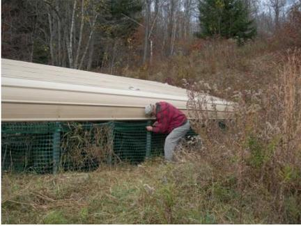
On October 25, 2013, Corey Richmond, Steve Szoke, Tom Yarnell and Carol Kafer did some maintenance work of the covers over the passive acid mine drainage (AMD) treatment intakes at Tunnels A & B on White Ash land in Sullivan County. The covers prevent algae growth, and the snow fencing keeps out the leaves. In the past, without frequent maintenance, the inflow pipes became clogged with algae and leaves. LCWA membership dues paid for
