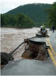
In September of 2011, a 500-year-flood cause a rupture in the petroleum transmission pipe line near the Wallis Run bridge.
